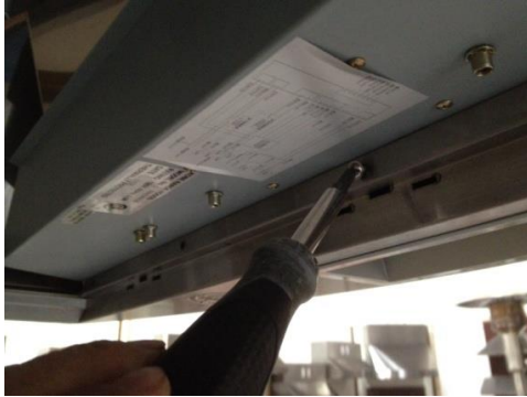
Figure 8: Halogen Lamp Transformers
