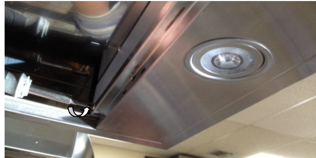
P4. Locate all the screws holding the LED Light Support Panel in place.
