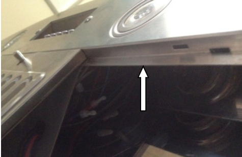
P1. First remove the baffle filters. If there is access to the back of the LED fixture, proceed to step 2. If there is no access please proceed to step 3.
